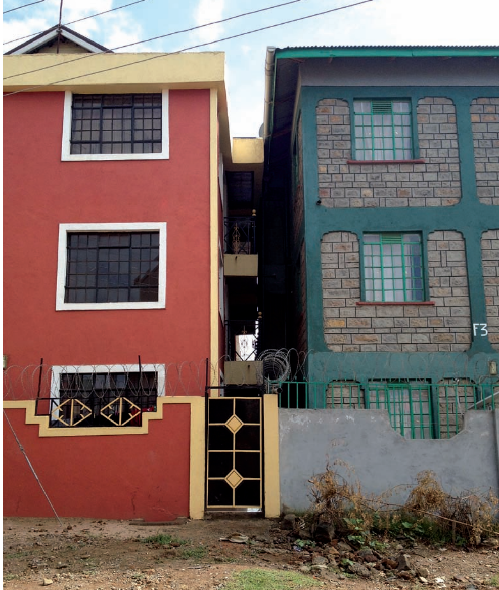
New apartment houses being built in Lolwe Estate, Kisumu (June 2014).
